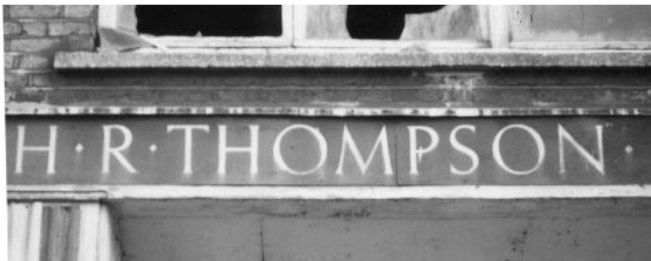
Fig. 14. Near the Museum of London; awaiting demolition.
